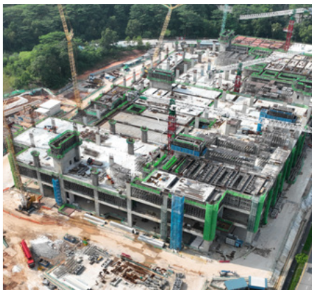
Construction progress update: Completed Level 3 slab.
