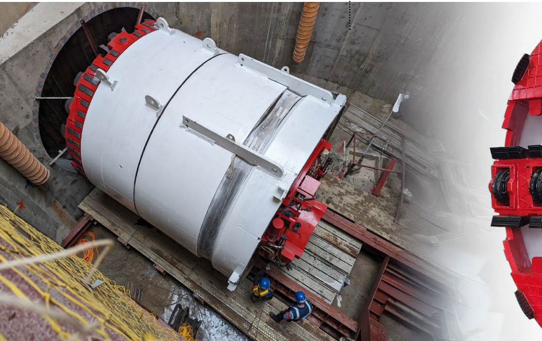
The middle shield of our Earth Pressure Balance Tunnel Boring Machine and close-up of the cutterhead.
