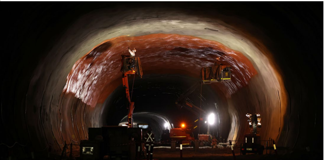
Waterproofing is a crucial step in ensuring the long-term durability and structural integrity of the tunnel, with paving, drainage and mechanical and electrical fit-out to follow.
