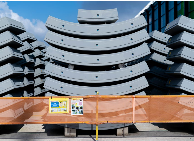
On the way to the shaft, we passed stacks of precast segments—each 1.4 m wide and 300 mm thick—which will be assembled into rings to form the tunnel lining as the TBM advances.
