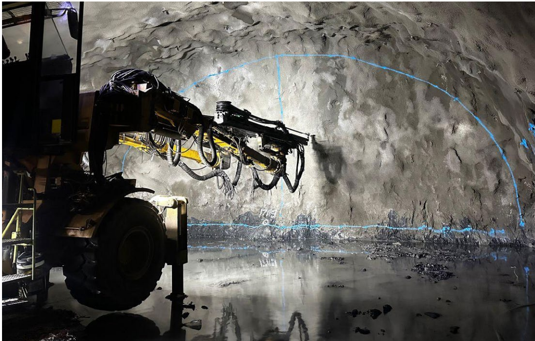
The face drilling rig (jumbo) follows the sprayed mark of the tunnel profile edge, which assists the drill operator. Each drilling cycle takes approximately five hours.
