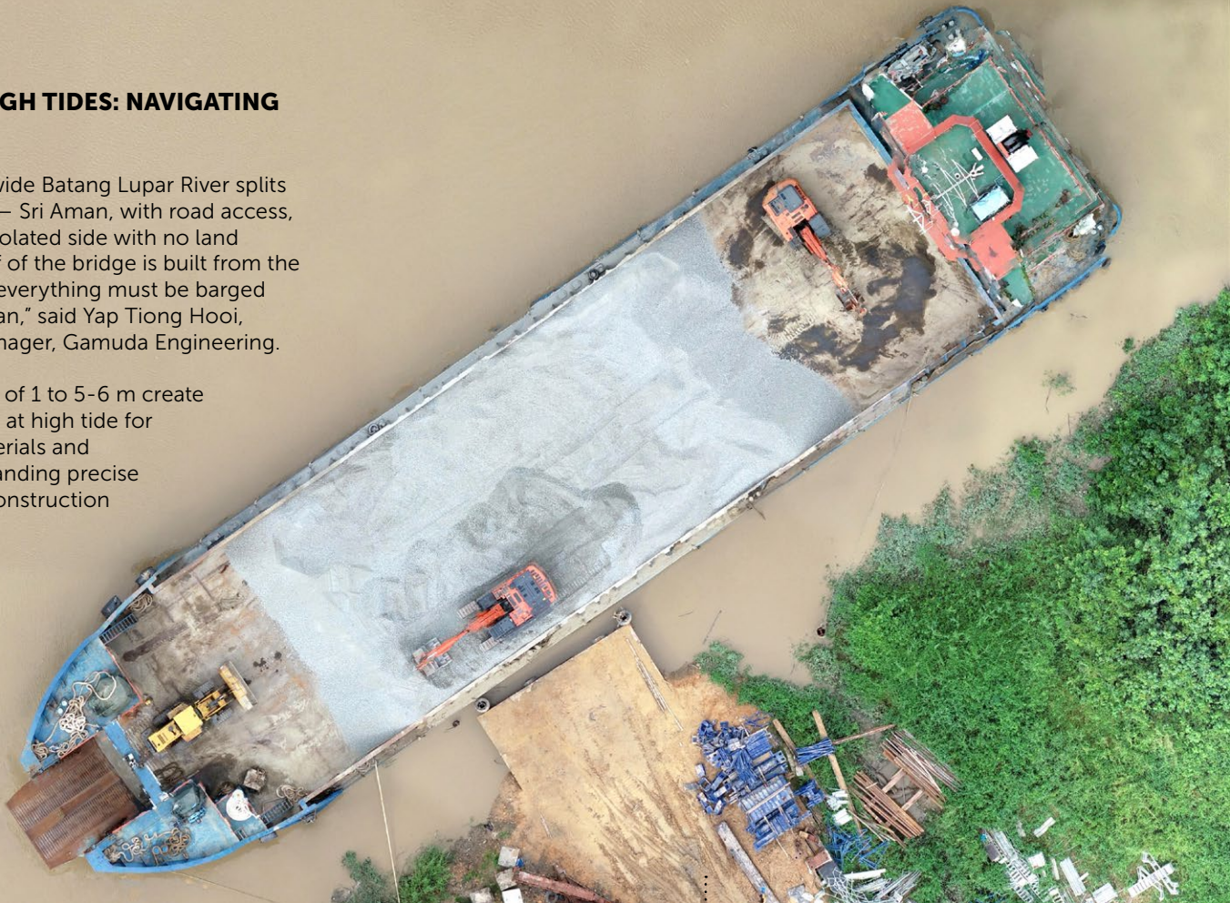
Barge arrivals are carefully timed with the tides to ensure efficient material delivery to the construction site — missing the window can delay construction progress.
