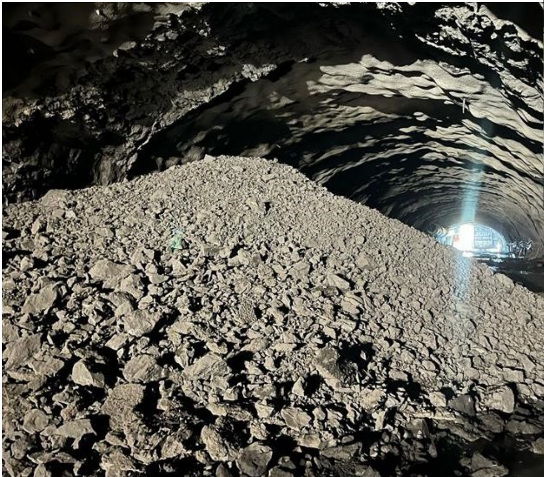
Breaking through Shephards Lane creates a direct passage through the 320 m tunnel.
