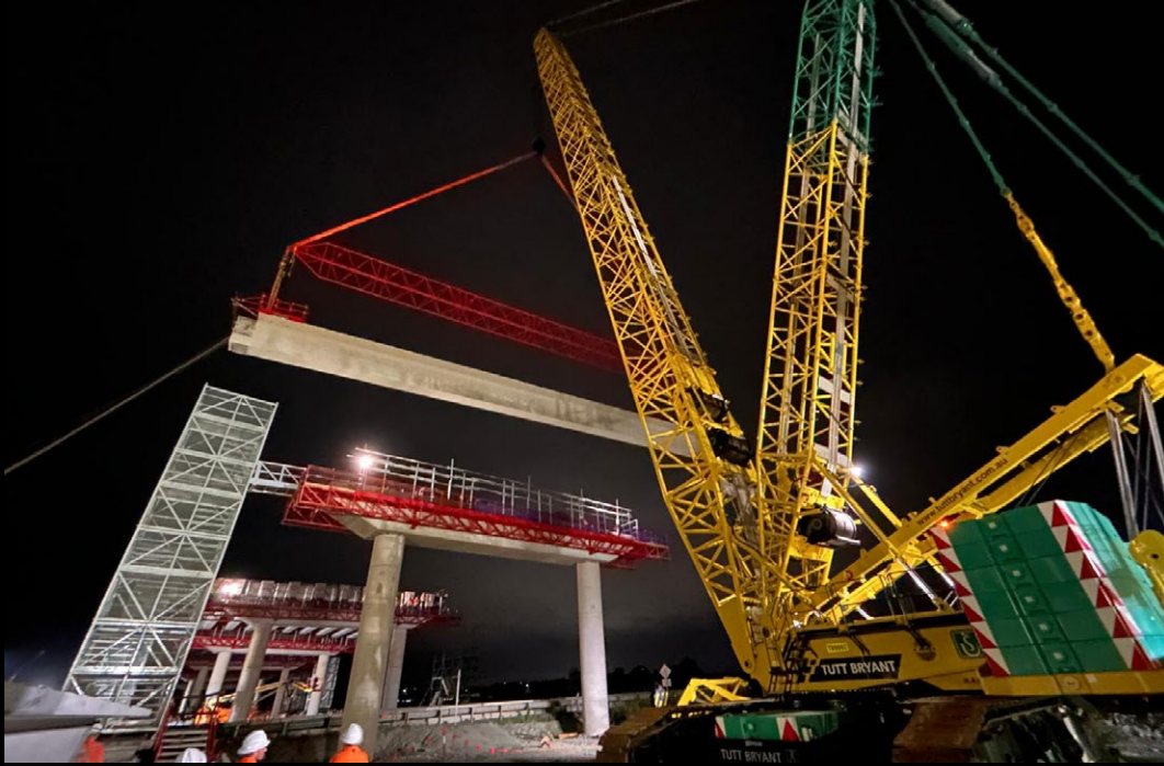
Prefabricated, enclosed access platforms on super-T girders (girder access platform). Providing safe access and edge protection for riggers and dogmen while eliminating the need to use elevated work platforms (EWPs).
