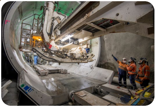
Compared to the traditional 'cast-in-situ' lining methods, the LEM is more efficient and provides a safer, stronger, economical and more precise way to build.
